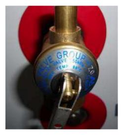
WARNING Fail to operate the relief value easing gear at least once every six months may result in the water heater exploding. Continuous leakage of water from the value may indicates problem with the water heater.
